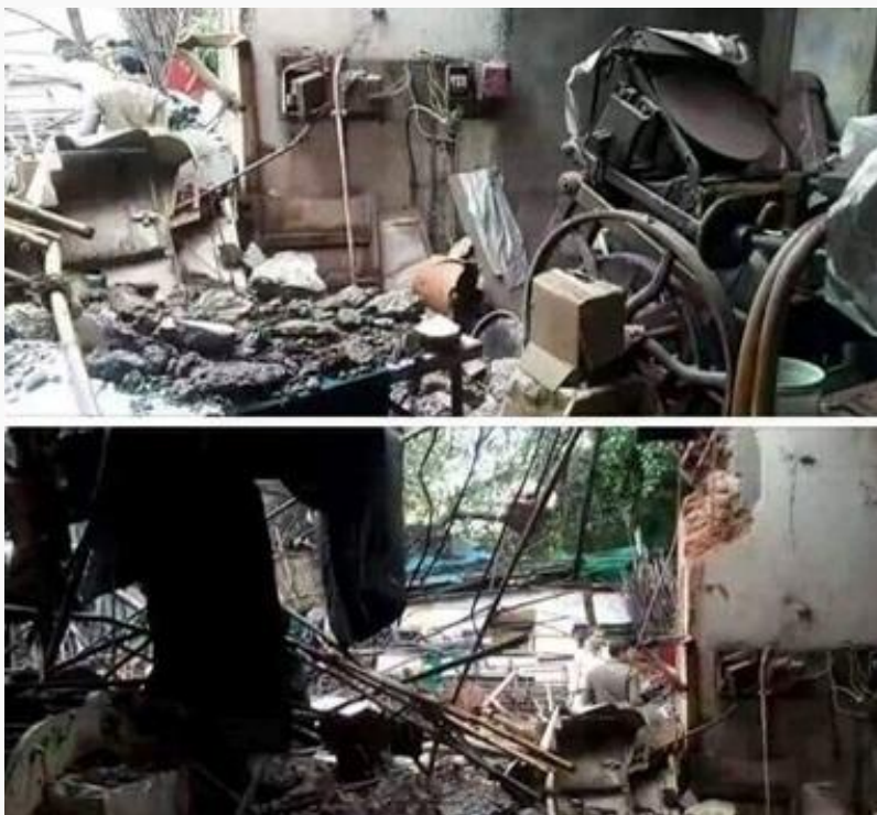
Figure 2: Pictures after Demolition on 25- 06-2016
