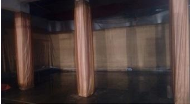
Inner View of the partly demolished structure
