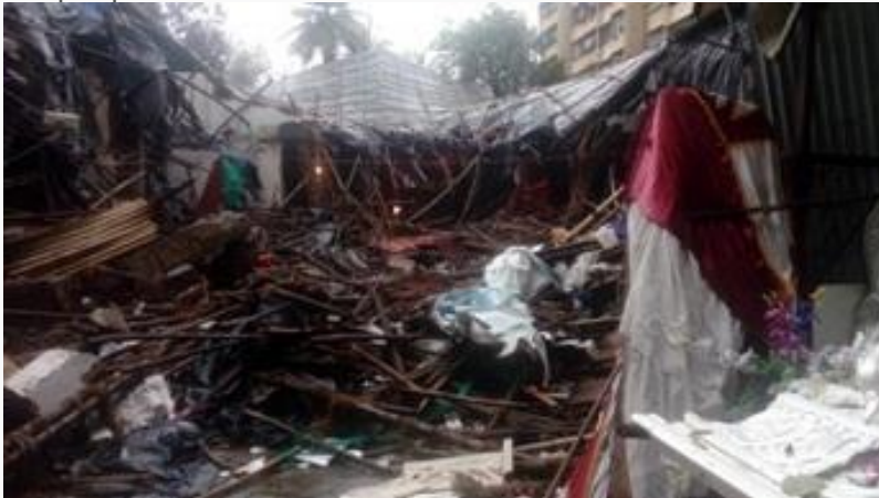
Front View of the partly demolished structure
