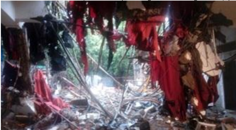
View from the remaining part of the structure
