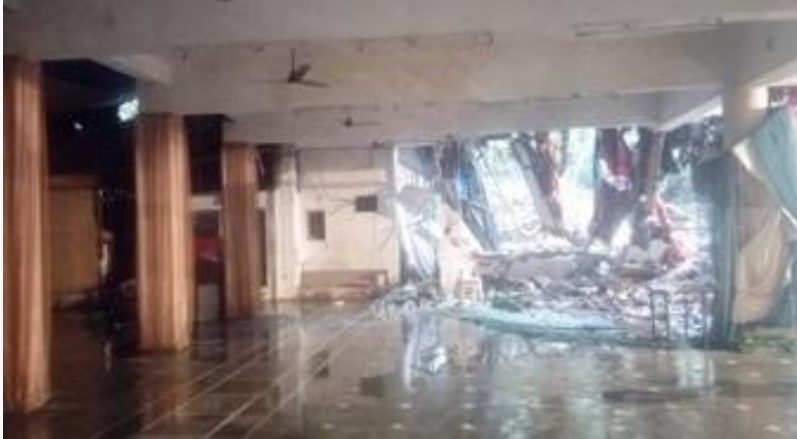
Inner view of the demolished structure
